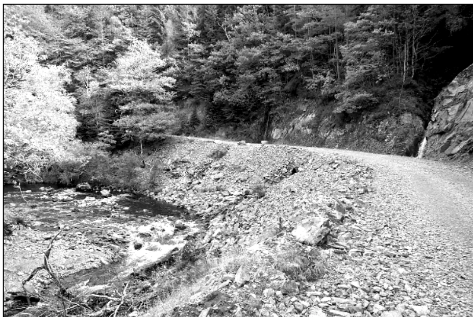
Fig. 14 Section of forestry road rebuilt after the 2001 flood.
