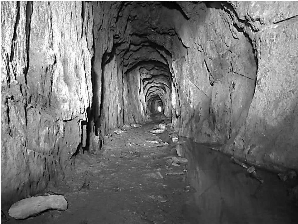
**Figure 151:** Adit tunnel leading to the underground waterwheel
